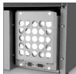
HEPA H14 filter and prefilter
